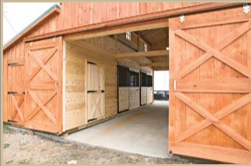
CENTER AISLE WITH NO LOFT
